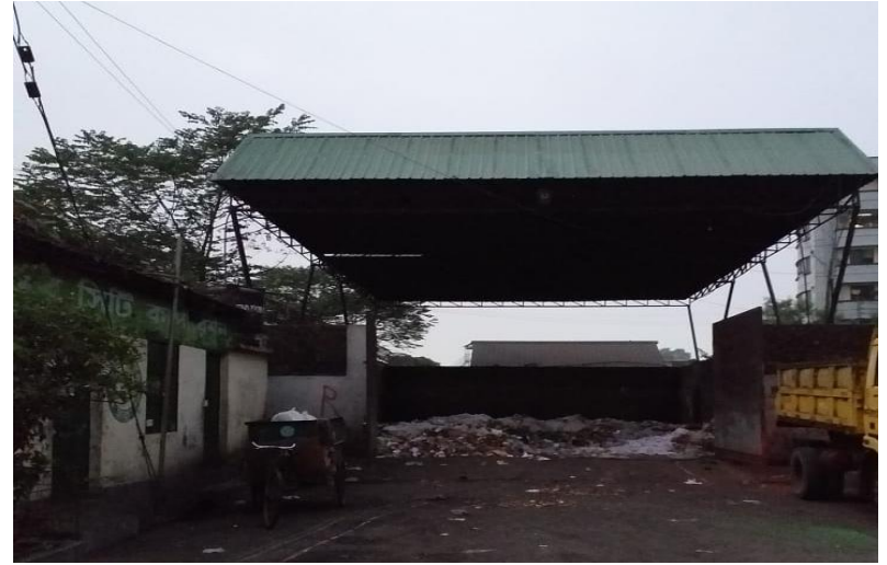
Figure: Waste storage in City Corporation selected location (Nikunja-2)
